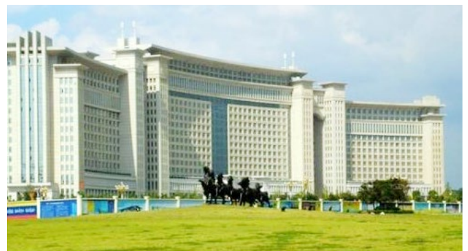
Government Administration Building
